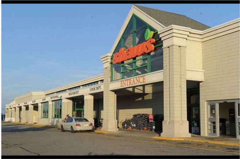
BUY PHOTO HIDE CAPTION The former Shaw's Supermarket in Fall River's South End shortly before it closed in 2013. [Herald News File Photo | Dave Souza]
